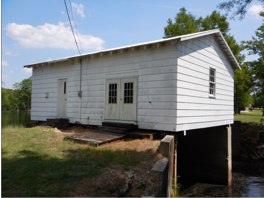
Photograph 13: View looking southeast at the ca. 1930 mill house.
