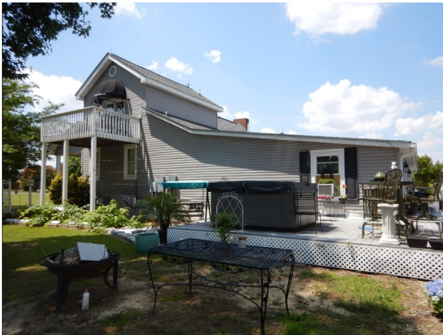
Photograph 3: View looking northwest at rear lean-to and extension.
