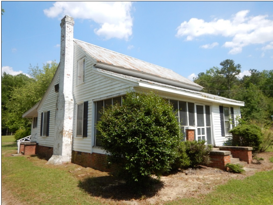
Photograph 8: View looking southeast at the 1929 residence on the Malcolm Jernigan Property.
