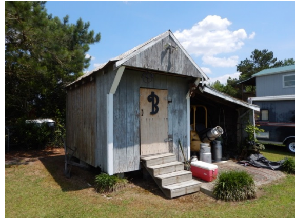
Photograph 7: View looking southeast at the frame storage shed.
