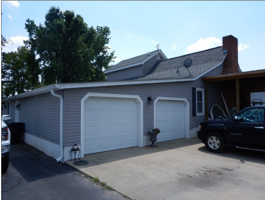
Photograph 4: View looking southwest at the modern garage addition.
