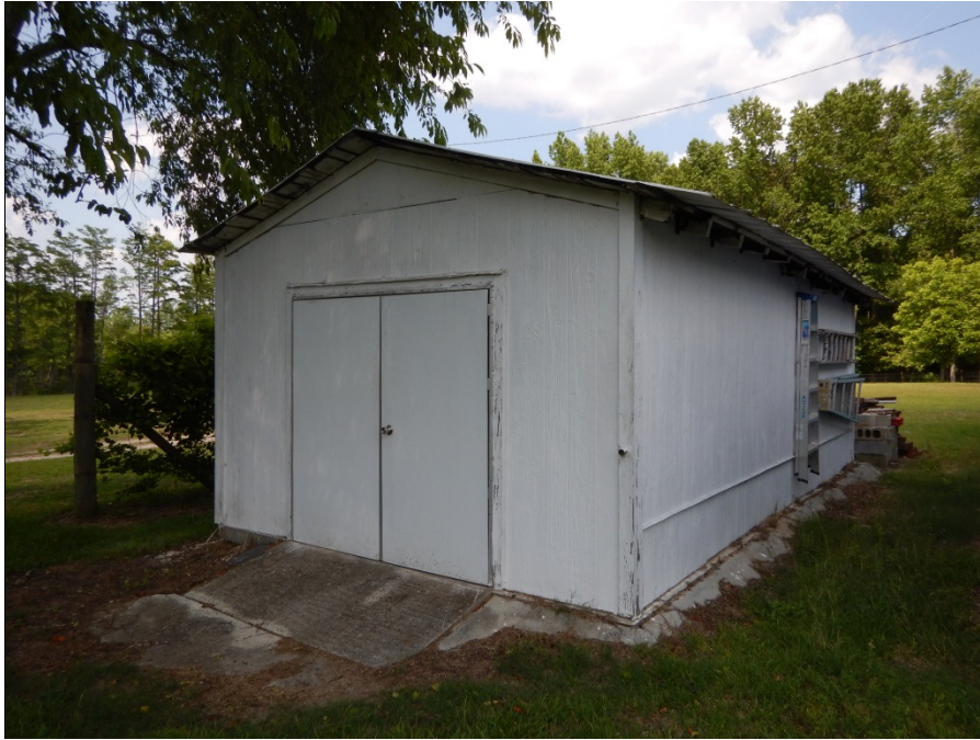
Photograph 12: View looking northeast at the frame shed to the east of the residence.
