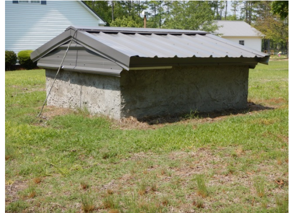
Photograph 18: View looking northeast at well cover.
