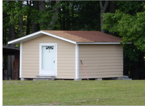
Photograph 16: View looking northeast at the modern shed.
