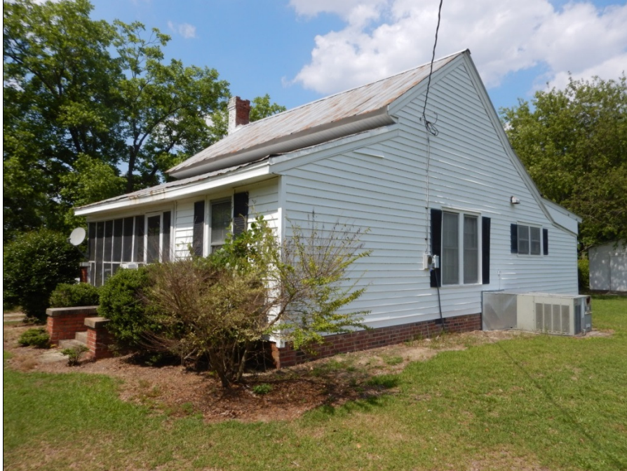
Photograph 9: View looking northeast at the 1929 residence on the Malcolm Jernigan Property.
