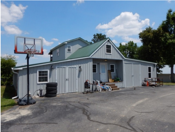
Photograph 6: View looking southeast at the stable/office building.
