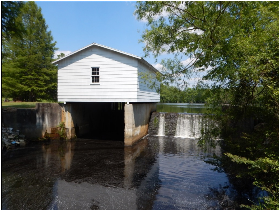
Photograph 14: View looking east at the mill house and dam at Jernigan Pond.
